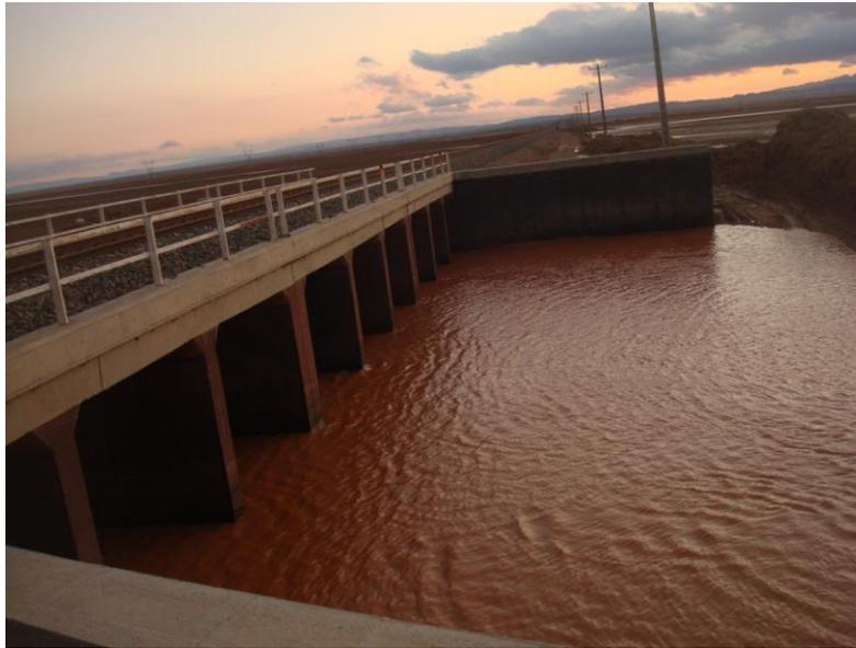
Figure 9: Accumulation of water under the bridge in Tabas railway
