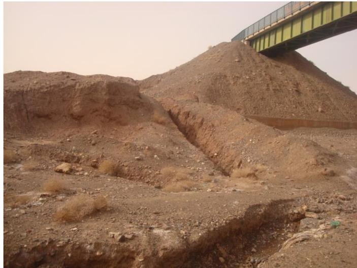
Figure 8: bed scour at bridge in Shadmehr to Torbat stations
