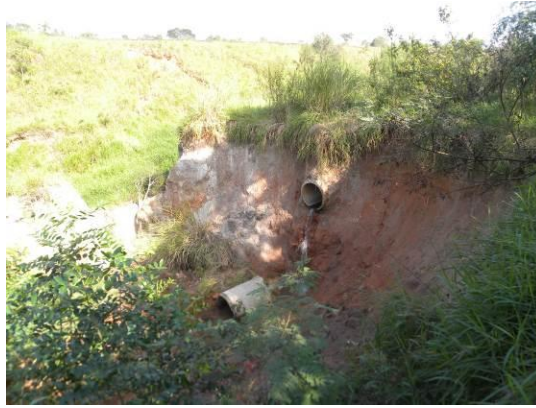
Figure 3 - Erosion ER-007 in June 2012.
