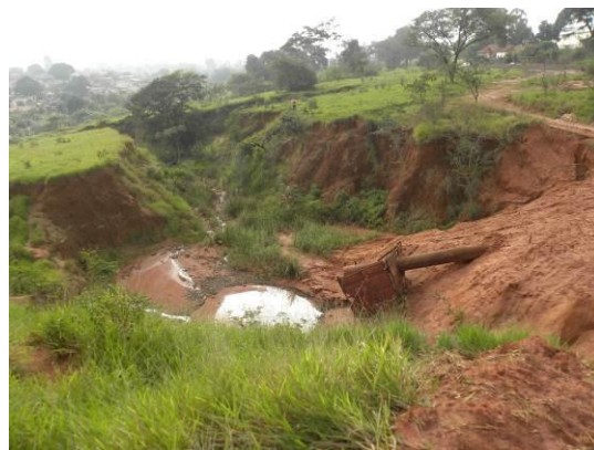
Figure 2 - Erosion ER-004 in June 2012.
