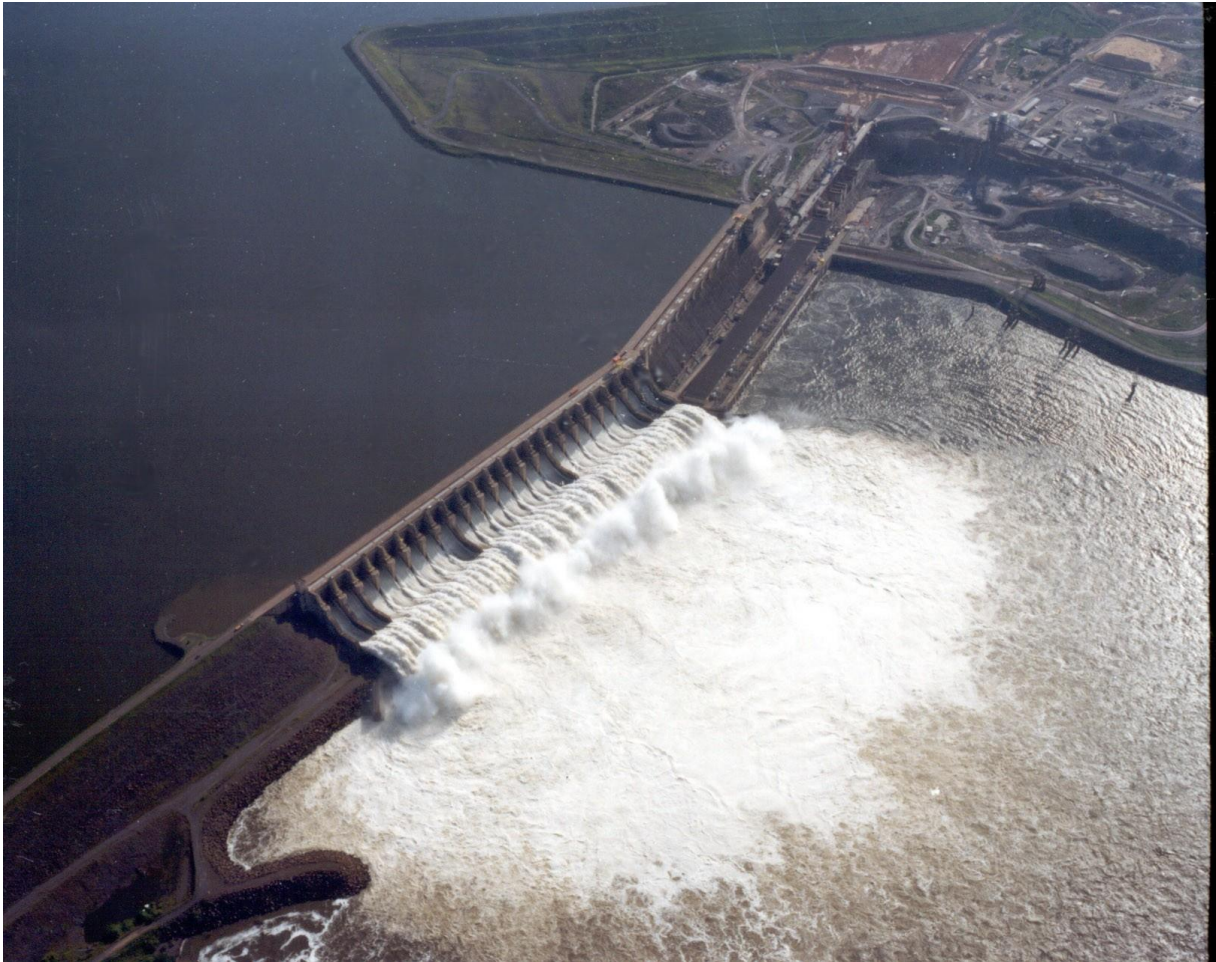
Figure 2: Opened outlets of the Tucuruí Dam.
