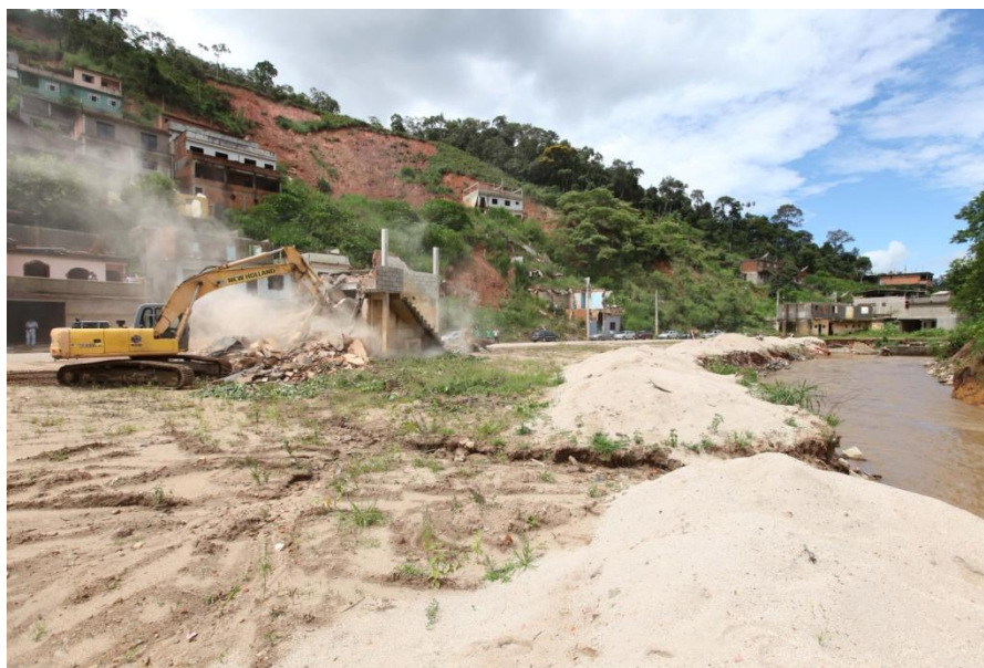
Figure 4: Demolition of residences lying in the floodplain with total occupancy restriction (Zone A) in the Região Serrana, Rio de Janeiro State ( http://www.rj.gov.br/ )
