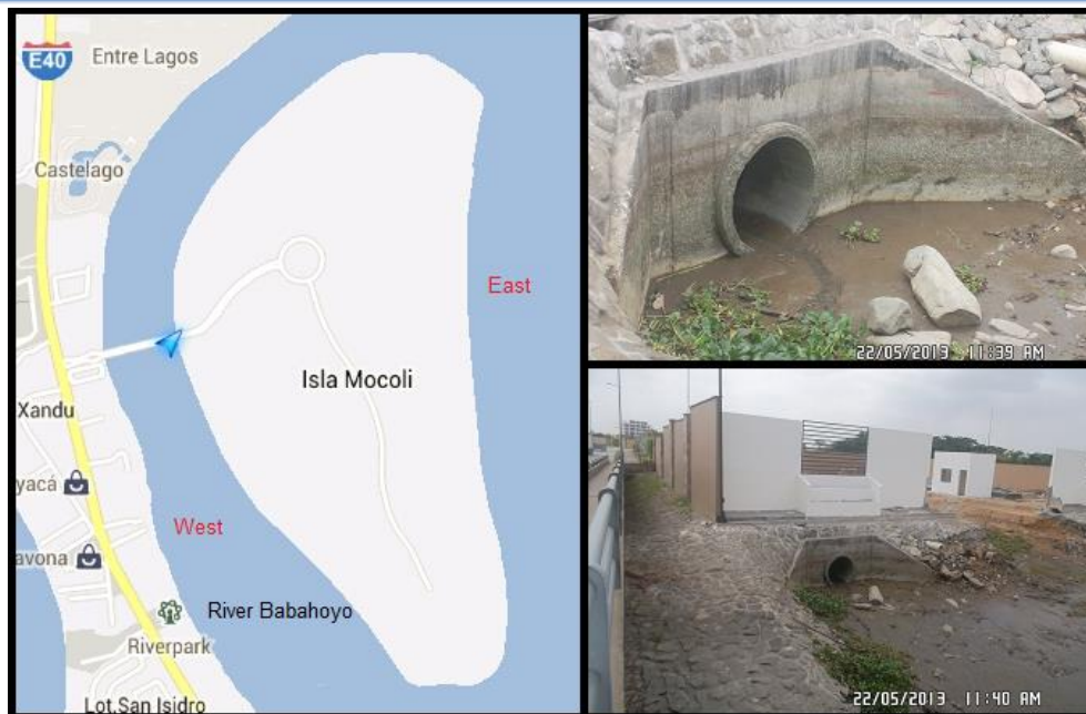
Figure 5. Sedimentation issues at the Mocoli Island western edge. How the sediments enter the main collectors can be seen as well, leaving remnants when the river levels decrease.
