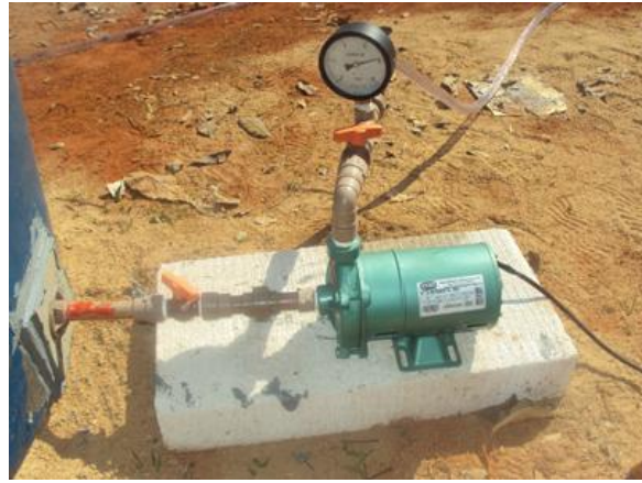
Figure 8: Turbo pump, pressure gauge and control records.
