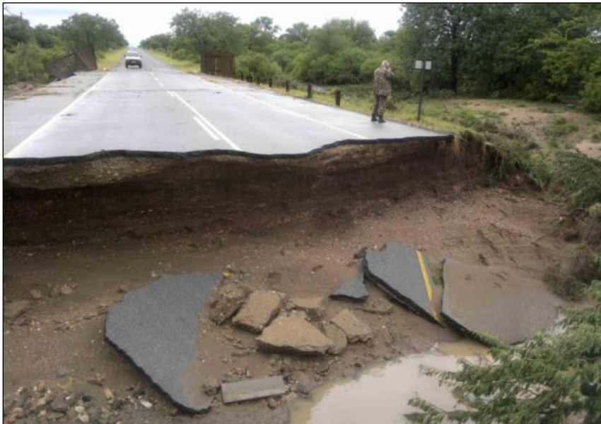
Figure 13(b) Road damage on access road to AFB Hoedspruit in Zandspruit
