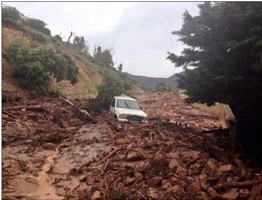
Figure 12: Road damage and debris at Chapman's
