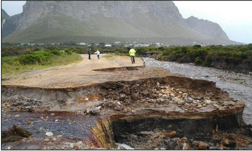
Figure 11: Road damaged by floods at Betty's bay
