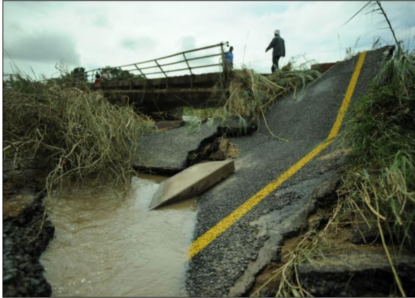
Figure 13(a): Road damage at Sandspruit River
