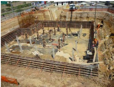
Figure 12 - Construction of Reservoir
