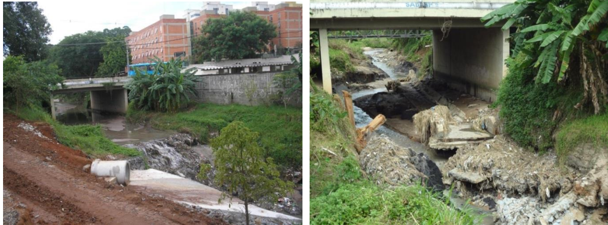
Figure 1.a - View of detention basin on Guadalupe Street, showing Senhorinha Creek, 05/03/2011.
