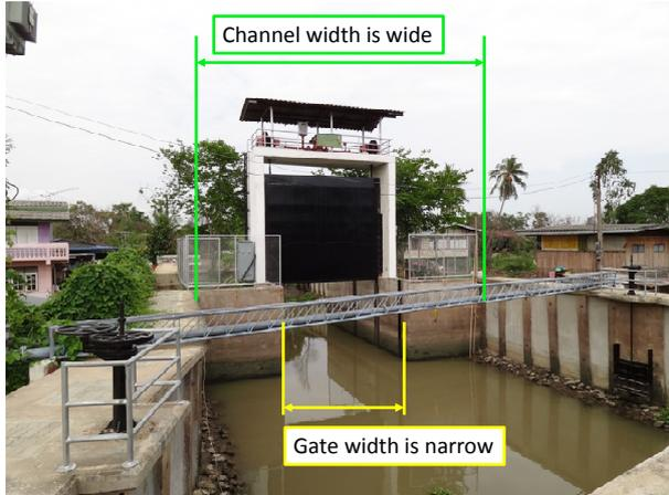
Figure 2: Gate in an Irrigation canal
