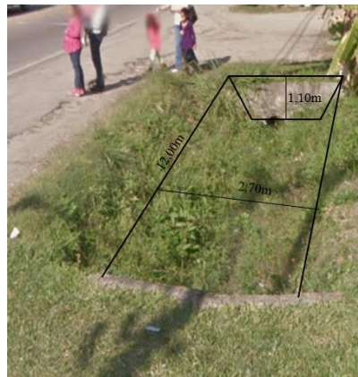
Figure 7 - Infiltration trench
