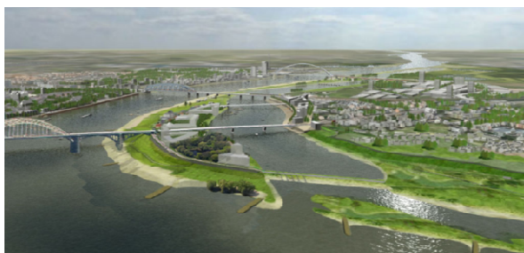
Figure 4a: Bypass Veur Lent (Nijmegen) accommodating 600 m 3 /s during extreme flood conditions (centre), in combination with an urban development project “Waalsprong”, consisting of 12,000 houses (right)
