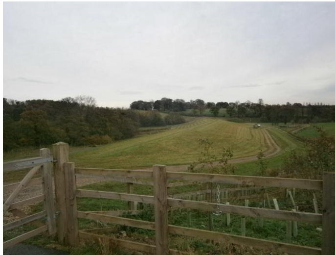
Figure 2: Birkby Nab dam.
